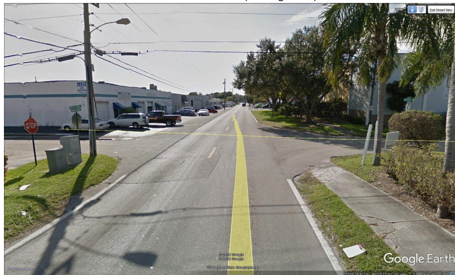
Park Road & SW 25th Street (Looking South)
