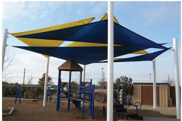
Fort Hood Army Base 3-Point Sail Joined HDPE
