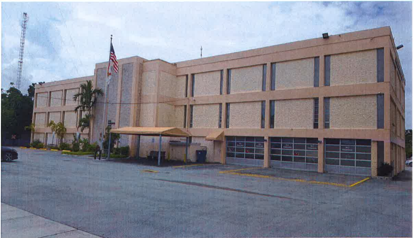
Town Hall Building (East Elevation)
