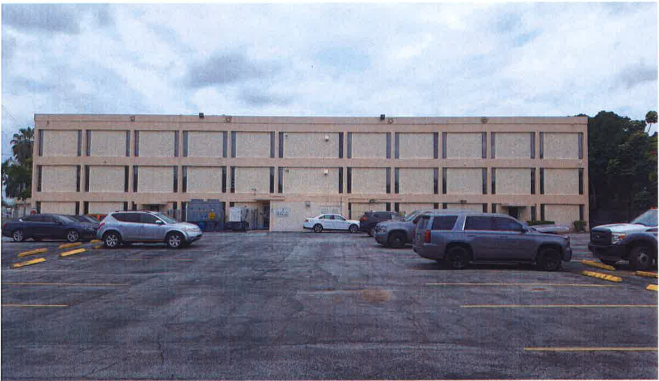
Town Hall Building (West Elevation)
