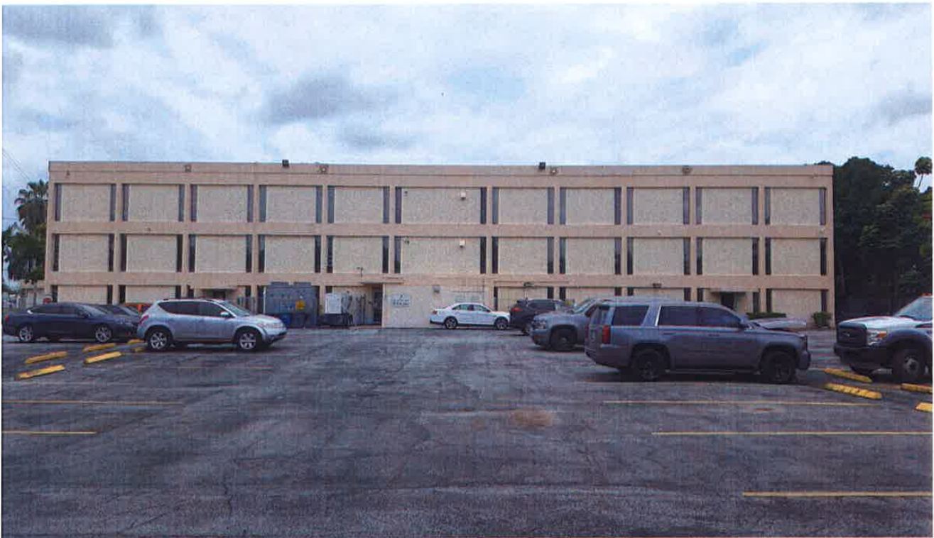
Town Hall Building (West Elevation)
