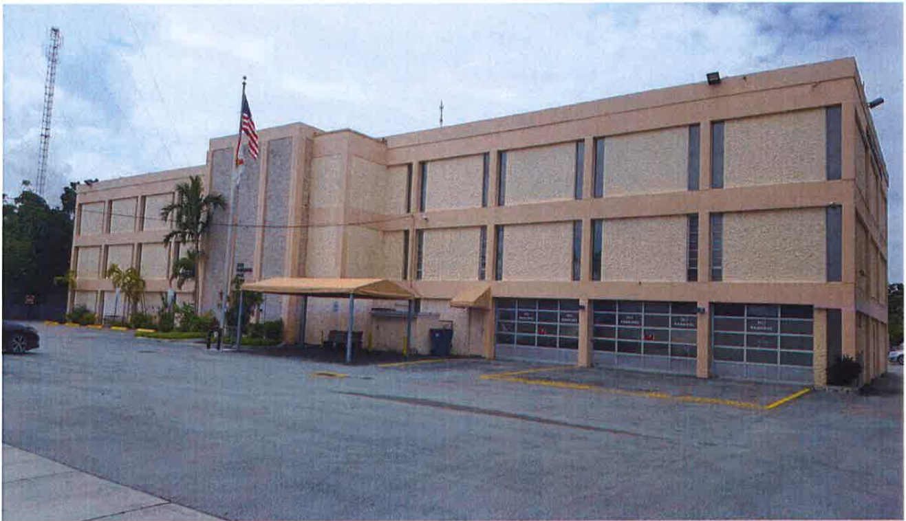
Town Hall Building (East Elevation)
