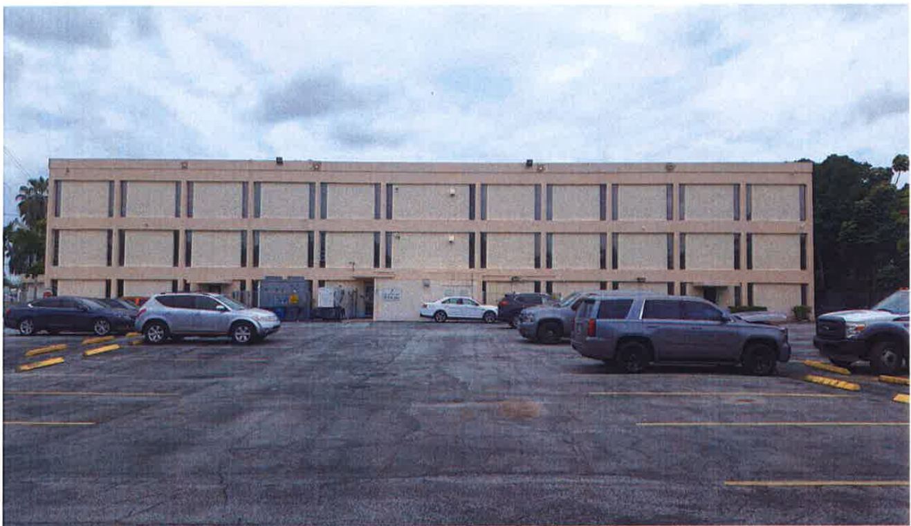
Town Hall Building (West Elevation)
