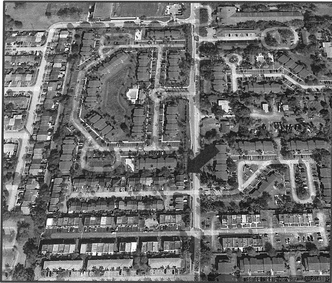
Figure 2 Aerial View of Subject Site. Source: Google Earth 12/10/2018
