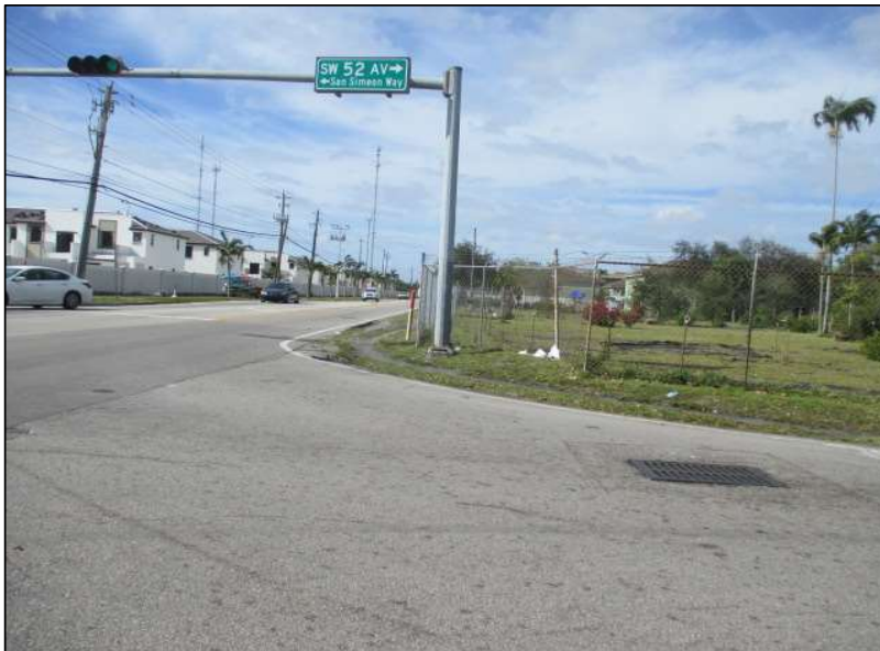
WEST ON COUNTY LINE ROAD
