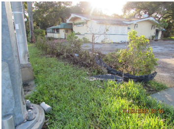
5590 W. Hallandale Beach Blvd - Replaced damaged hedges
