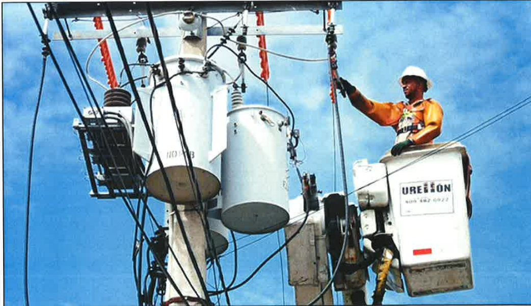
Utility shutoffs will be suspended for Florida residents.
