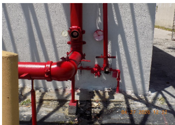
2500 SW 30th Ave - Backflow preventor leak repaired
