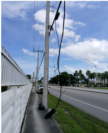
W. Hallandale Beach Blvd & SW 52nd Ave (R.O.W.) - Comcast down communication line was repaired
