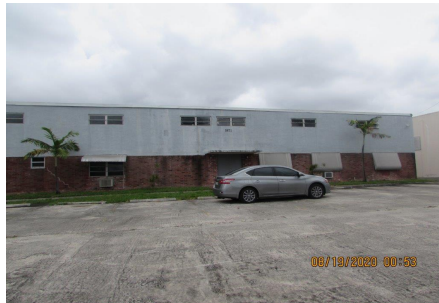
1971 S. Park Road - Clean and Repaint building
