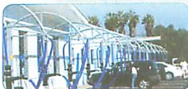
Vacuum booms with dual drops without canopies
